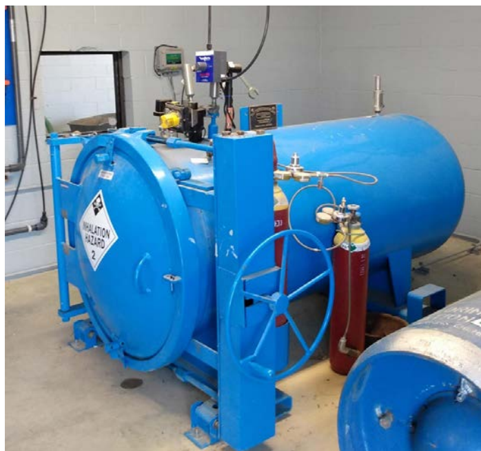
ChlorTainer's failsafe valve is powered open using nitrogen and electricity. If the power is lost, the failsafe valve will cycle closed, and will automatically cycle open when the power is restored.
