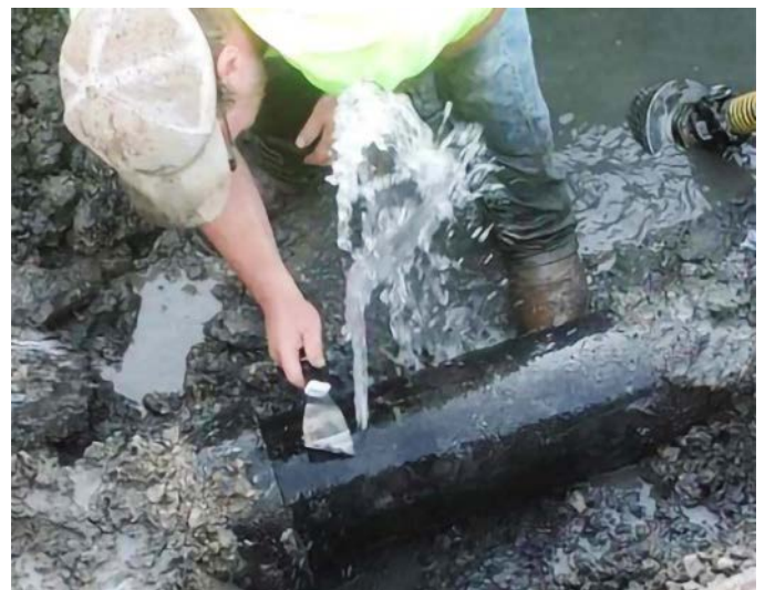
Cody Springston scrapes the water main before installing a repair band.
